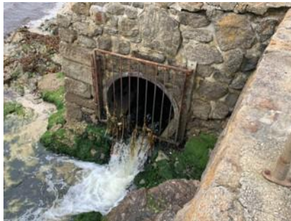
Swanpool stream at beach, end of culvert
